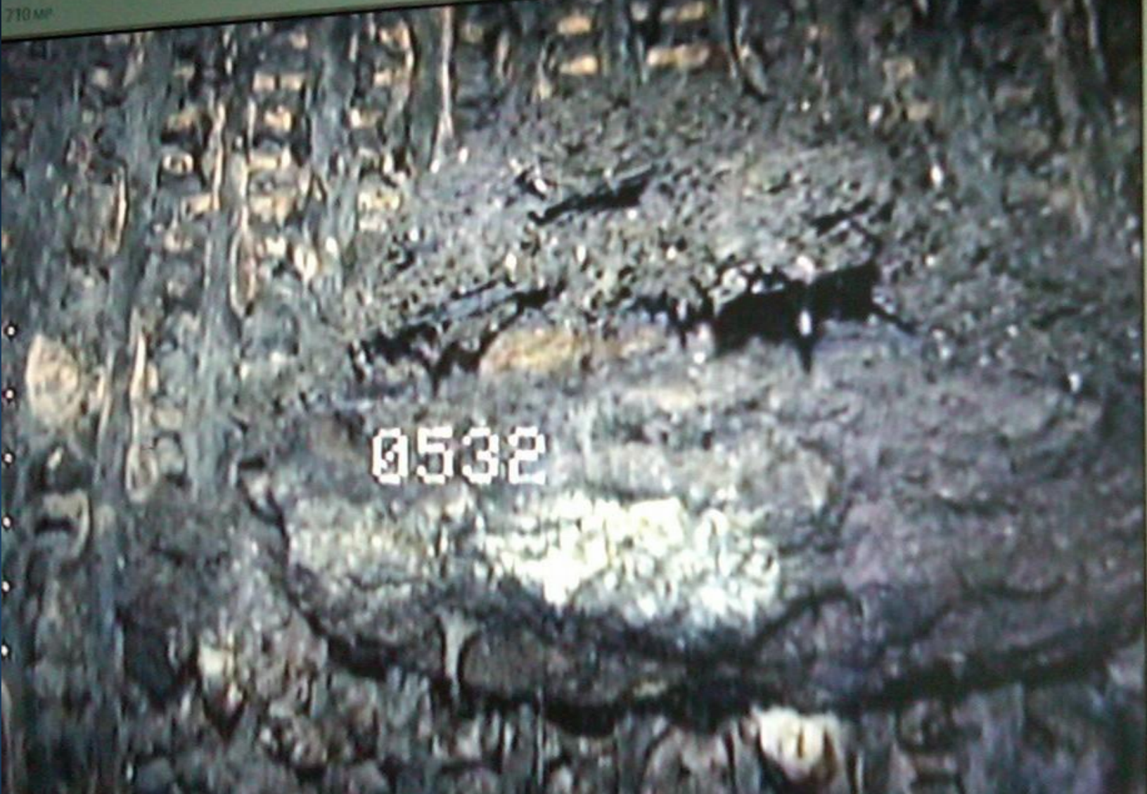
Well 4-55 – Scaling (precipitation) with nodule Wire-wrap screen at 532' – 07/27/2010
